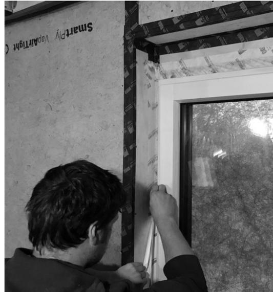
**Figure 5. Windows installed in the dry behind the wrap during heavy rain.**
