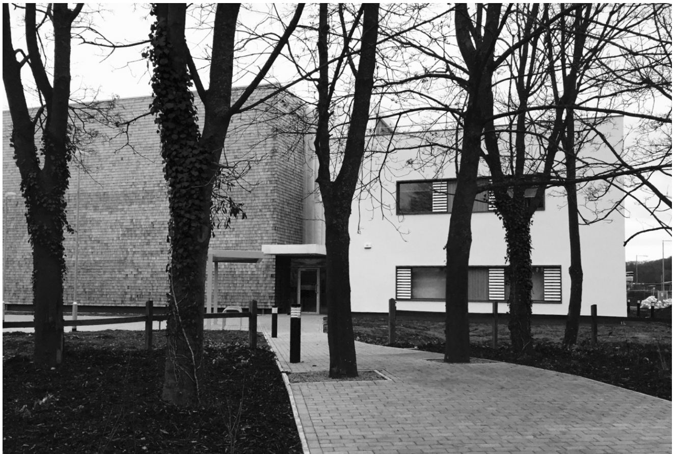
Figure 1: Hereford Archive and Repository, West elevation.
