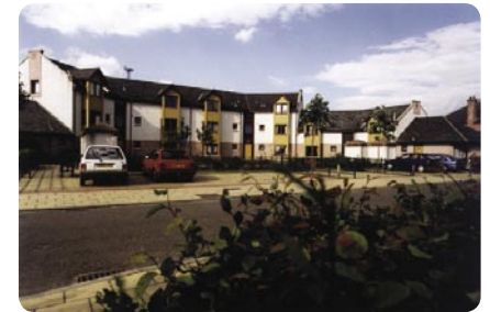
Leslie Court Fairfield, Perth - Fairfield is shortlisted for the World Habitat awards. The Sunscoop on phase 7 is based on permaculture principles. The development includes several passive design items. The whole project was delivered without subsidy at yardstick costs. (Gaia)
