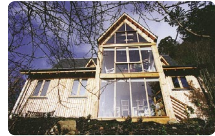
Tressour Wood House - House of the Year 1993 - the unheated conservatory was incorporated into the stairwell - mezzanine at the landing. This meant that the temperature regime could vary according to outdoor climate and the sitting area would only be used when comfortable. (Gaia)
