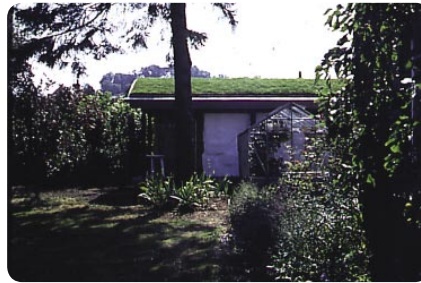
Dunning - Straw bale office in Perthshire - with a turf roof at client insistence - conceded when they agreed to grow strawberries on it. Membrane is latex based. (Gaia)
