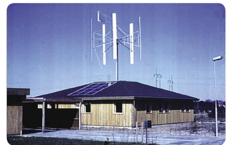
Windmill House Skive, Denmark - the house was one of 9 different experimental eco-technology houses built in 1977. The windmill became redundant very soon after commissioning due to excess vibration in the house.
