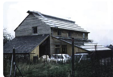
The Granada House - Built in 1975 as the focus of a television series "House for the Future" - With 13 programmes @ one technology a week, the house ended up looking like a Christmas tree. The solar roof contributed 2% to the annual energy input - with heat recovery from the cooker outstripping everything else - because the building was superinsulated. (Howard Liddell was a consultant to the programme and worked on the house with the TV team. Architect Don Wilson).
