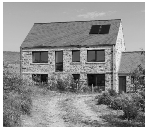
Figure 1. Steel Farm Passivhaus.
