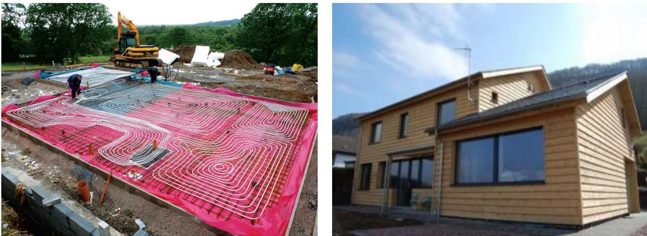
Figure 4: Laying the underfloor pipework in Taliesin Passive House (left); finished house (right)
