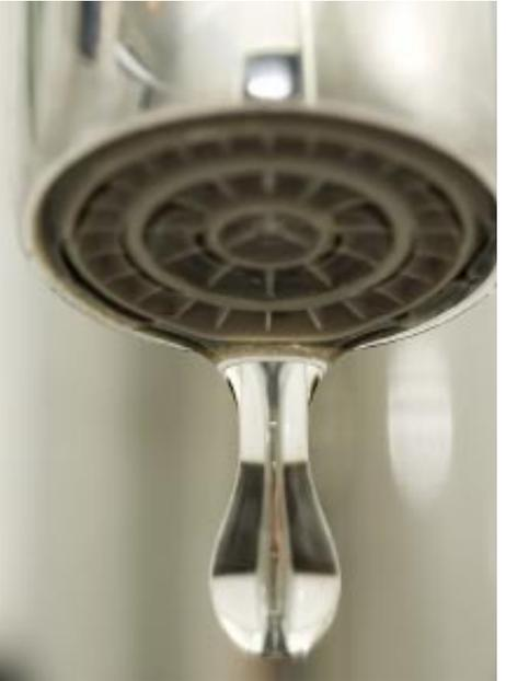
Regular maintenance is crucial if savings are not to be lost through leakage or malfunction. Even slow leaks can lead to significant amounts of water being lost if they are not fixed promptly. Suspected leaks are best detected by checking the water meter overnight or when a building is unoccupied.
